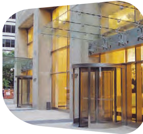
55 Water Street, New York, USA.
